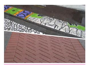
Inlaid thermoplastic pavement markings [above] can be used to create custom colorful graphic patterns that last longer than typical road markings. Imprinted hot mix asphalt crosswalks [below] can mimic brick or other masonry patterns, but are much more economical and durable.
